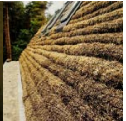
Seaweed Insulation Insulation Infill. Eradicated seaweed, ib Ungermund, Denmark.
