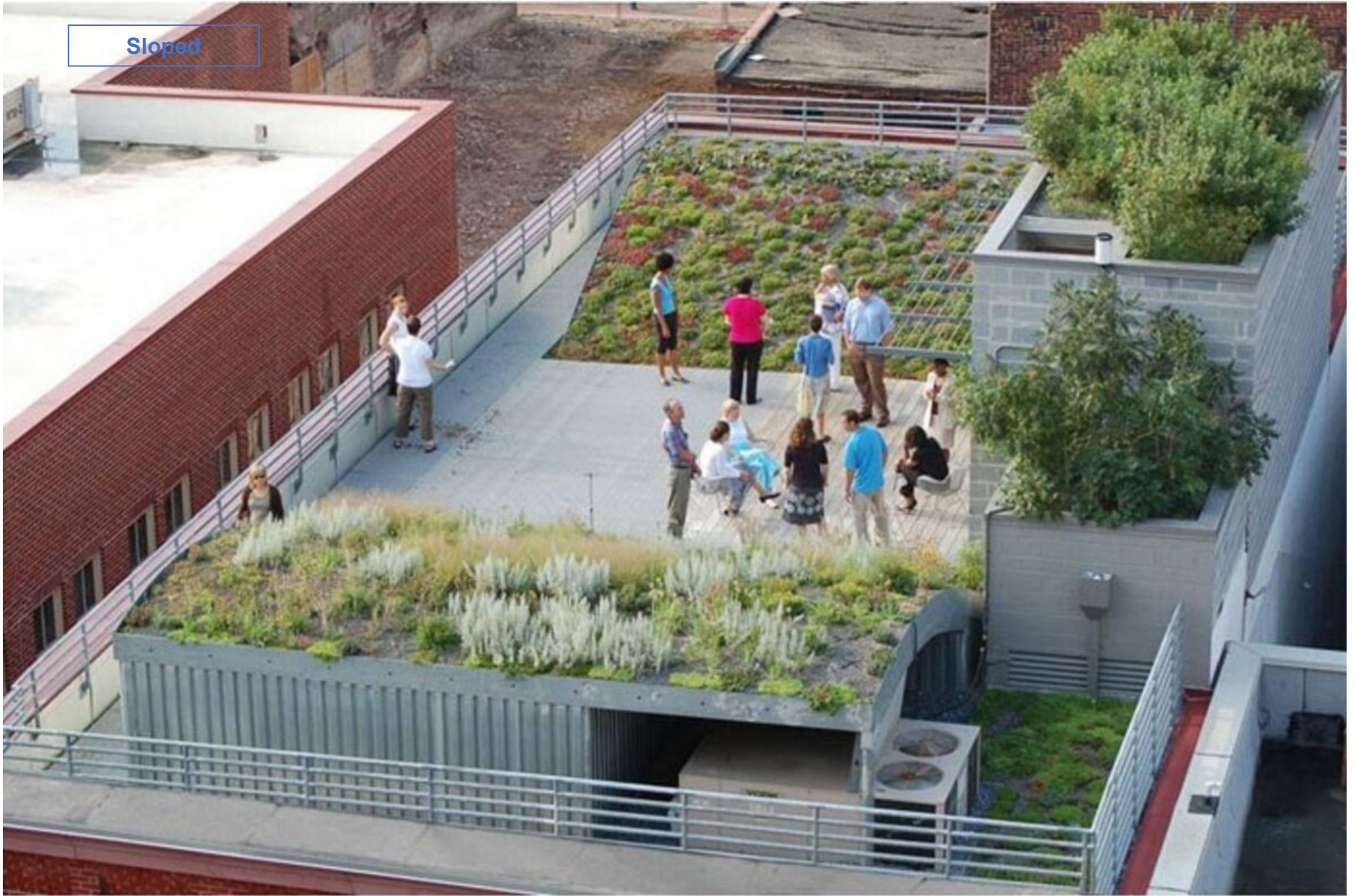
ASLA Headquarters Green Roof
