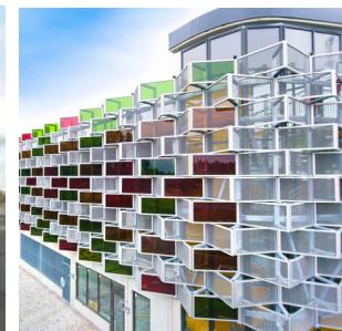
Solar parking deck, Sweden
