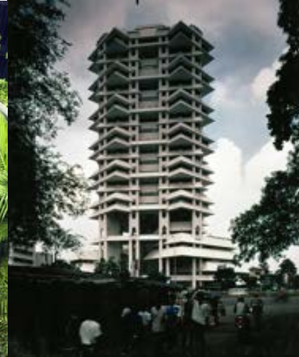
Wisma Dharmala Tower Jakarta, Indonesia | Paul Rudolph
