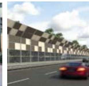
Solar acoustic barrier, Canada
