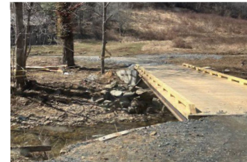
Figure 2. The completed construction of a temporary bridge at one of the many bridge sites. Our bridge design is similar to this bridge which includes a gravel-laden gravity foundation. The bridge is donated and built by two churches from coastal region.
