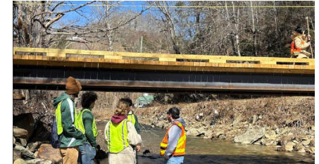
Figure 3. The side view of the temporary bridge shows the characteristic steel girder bridge with wood decking. The elevated bridge height is to prevent from potential future flooding that may be congested by the bridge height resulting in backwatering upstream watershed.
