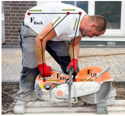
Figure 1. Masonry worker injury prevention study
